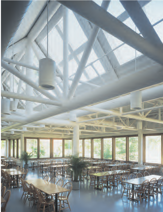
Figure 10: Toplighting with skylights, clerestory windows, or tubular daylighting devices helps to bring daylight deeper into rooms. Toplighting is feasible as a supplement to sidelighting. Photo: Velux America.
