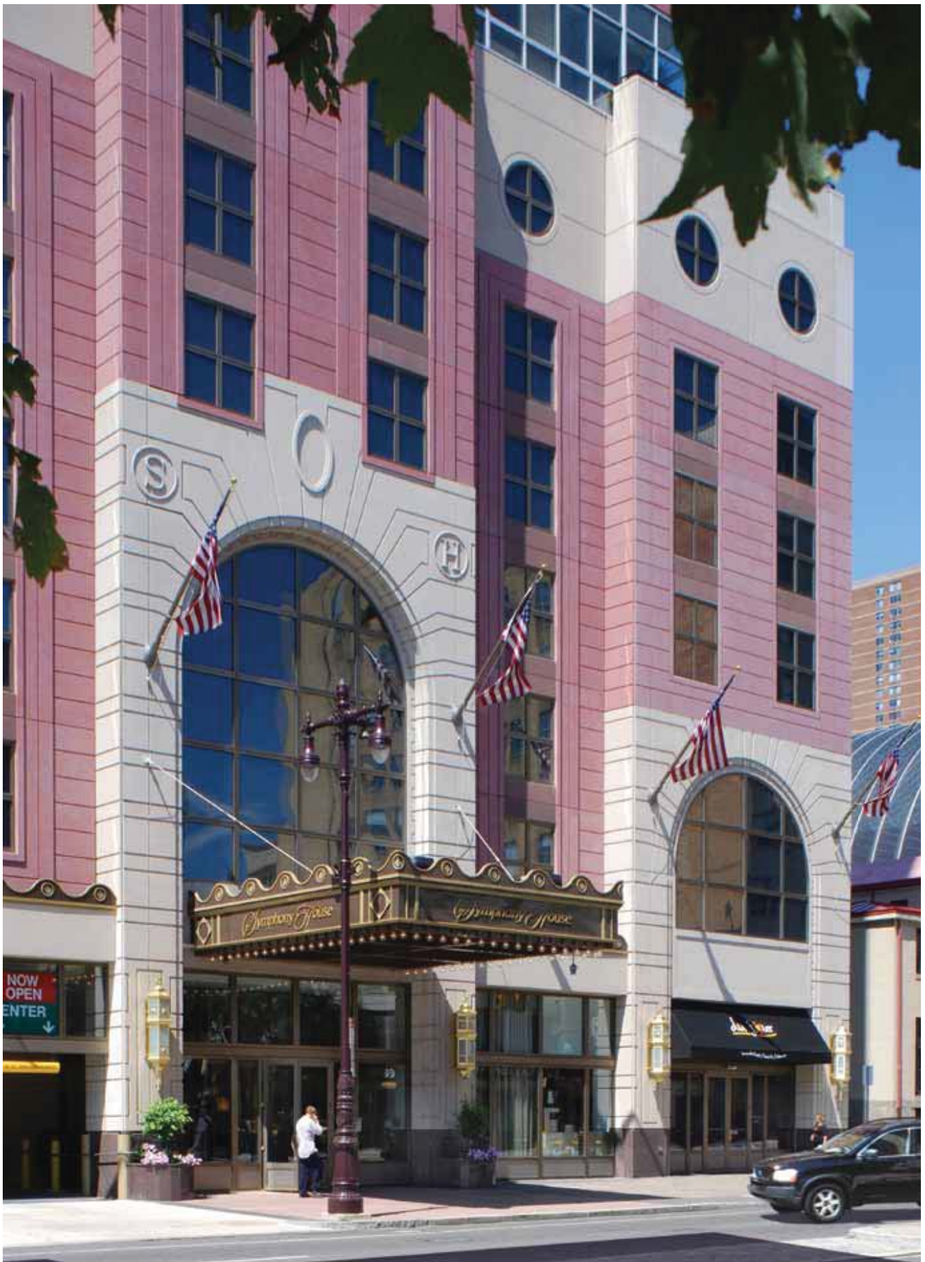
The 32-story Symphony House condominium tower in Philadelphia combines carbon-fiber reinforced architectural precast concrete panels with “punched” windows to leverage the use of daylight while providing sunlight control and high energy efficiency. BLT Architects served as the architect and interior designer. Photos: Michael Ytterberg.
