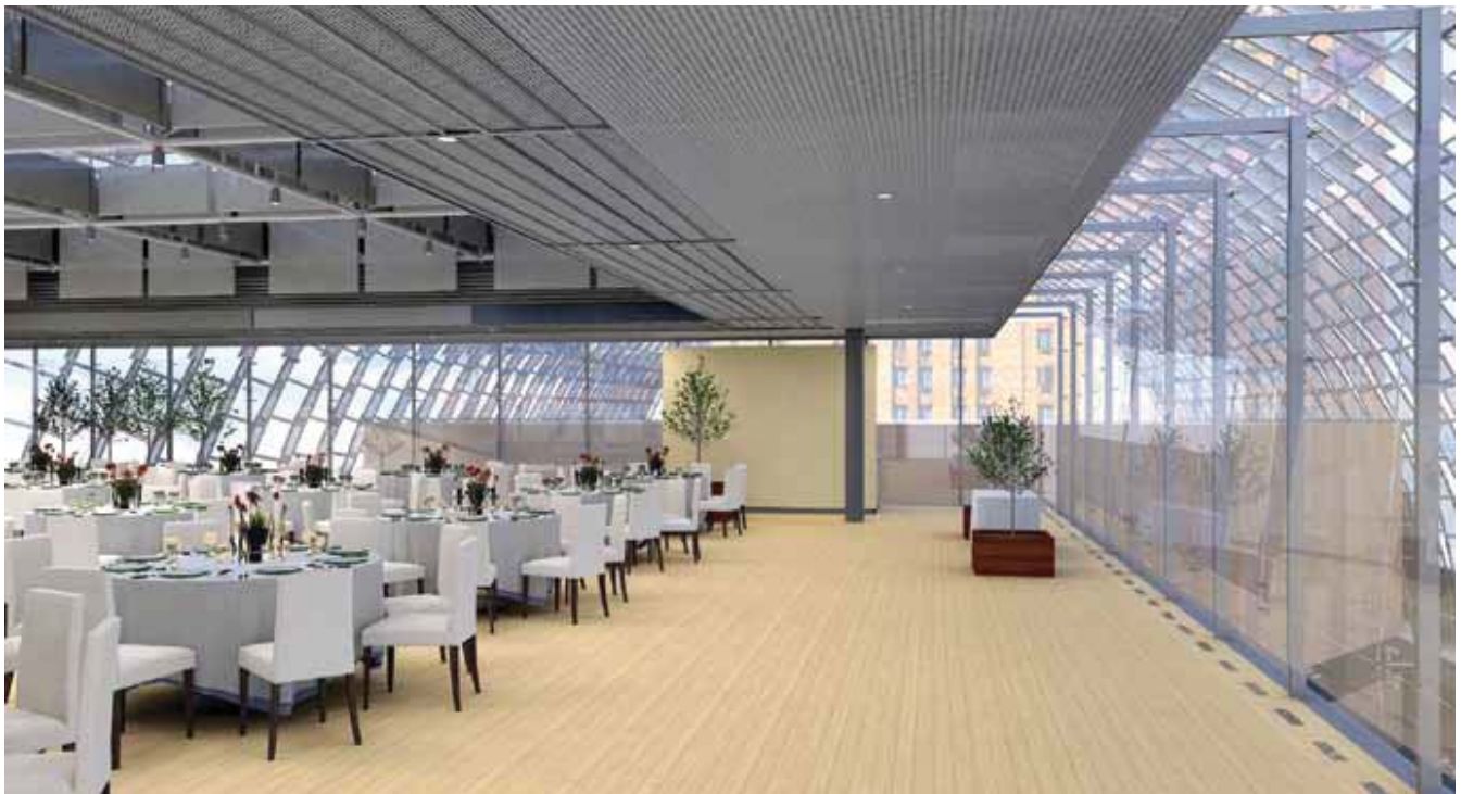
The Hamilton Gardens social space atop Philadelphia's landmark Kimmel Center for the Performing Arts is being enclosed in a carefully crafted glass and metal enclosure that will modulate environmental conditions after its original glass-roof design proved too difficult to control. BLT Architects served as the architect and interior designer. Rendering: BLT Architects
